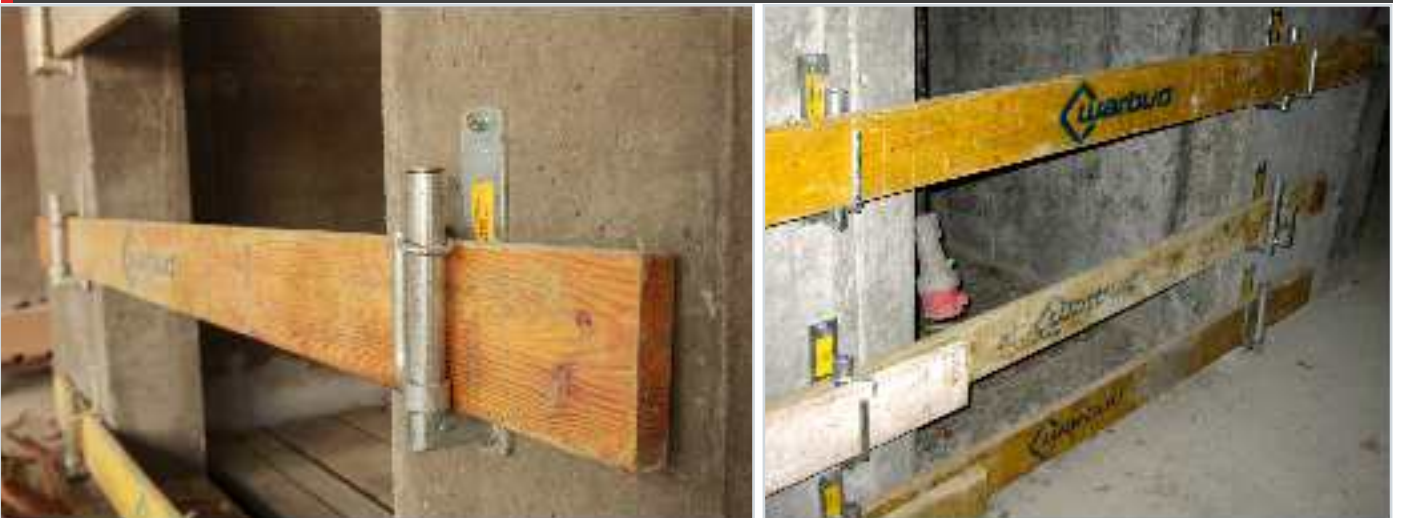
Elevator shaft grip
