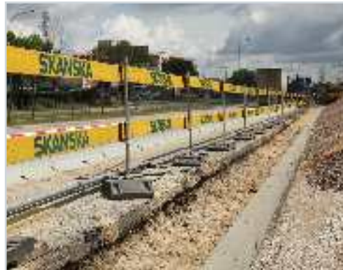
SECUMAX system, rebuilding of the road in Warsaw
