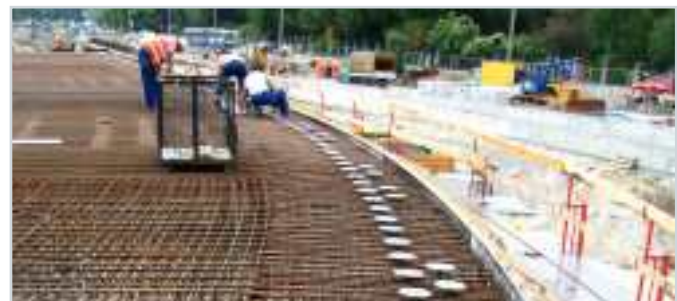
The disc anchors type I embedded in bridge concrete reinforcement
