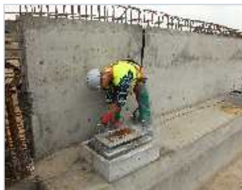
Mounting of the construction bearings, construction of the road S8
