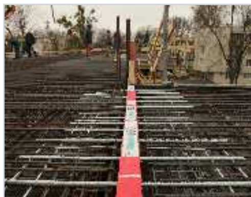
Installation of balcony connectors on the construction site
