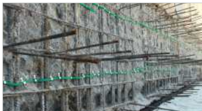
Using of the injection hoses P-100
