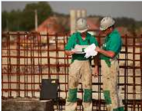
Construction bearings, construction the A2 motorway
