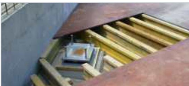
Formwork panels bridge with elastomeric bearings
