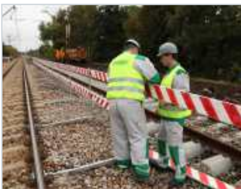
Installation of protective barriers SECUMAX RAIL on the trackway
