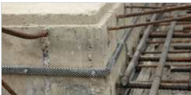
Example of use FORBENT tape type S
