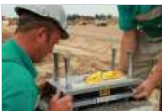
Formwork panels bridge with elastomeric bearings
