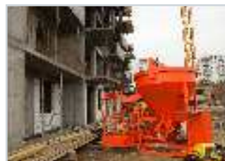
Transport of container for concrete
