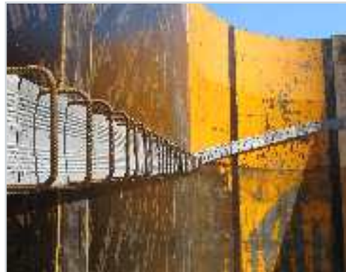
Concrete reinforcement banded BINDAX, construction of the parking in Cracow
