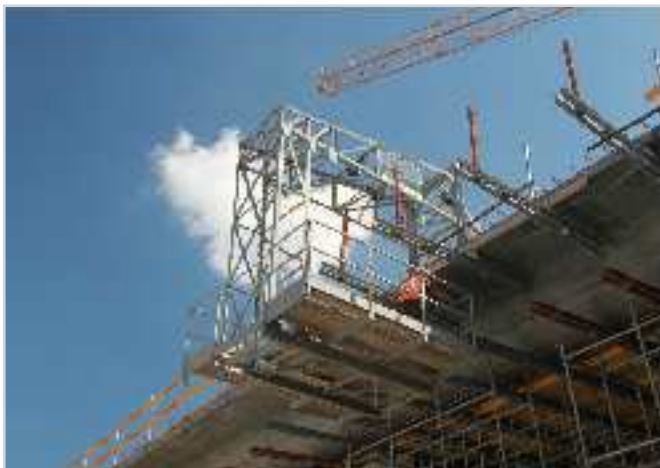
Mounting trolley during works on the viaduct
