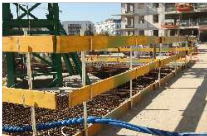
Application of the Secumax system on the construction of the housing estate
