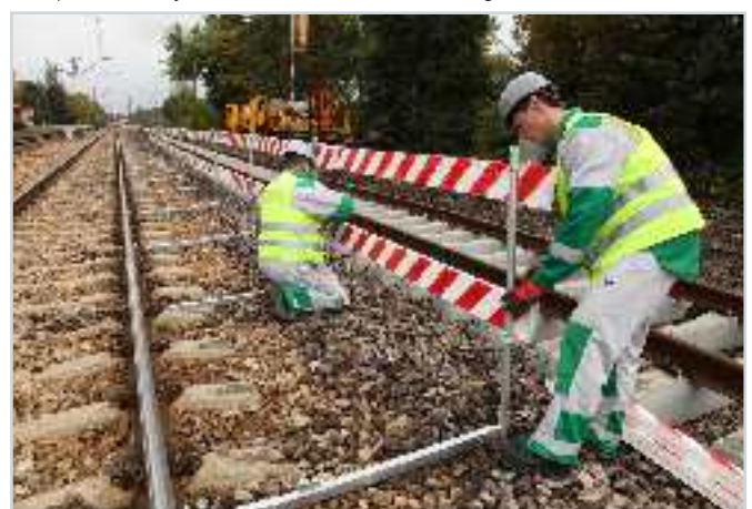
Assembly of the SECUMAX RAIL protection system on the trackway
