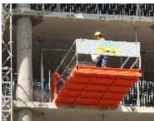
Unloading platform, construction of skyscraper in Warsaw
