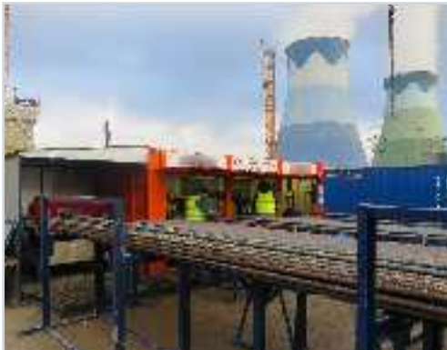
Production of BARTEC connections, construction of the power station in Opole
