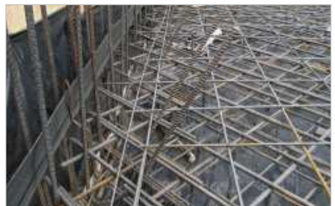
Using of the anchoring loop
