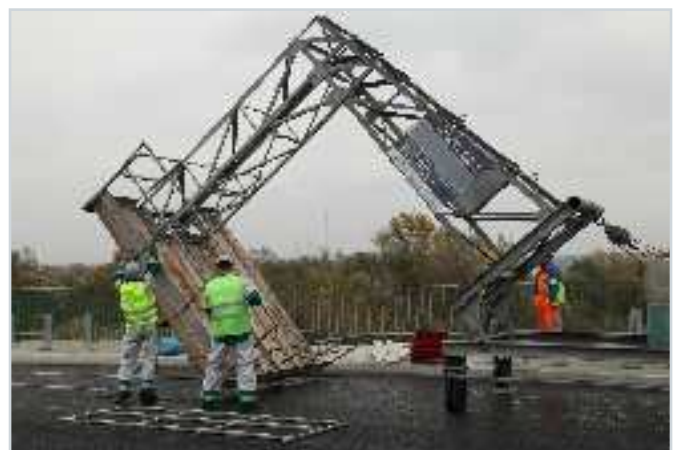
Mounting the trolley on the bridge
