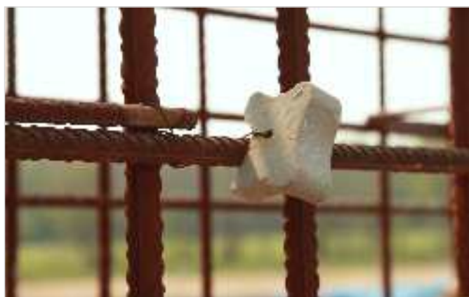
Using of FB bone point spacers
