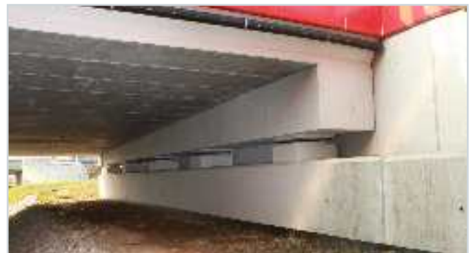
Elastomer bearings on the bridge over the A2 motorway
