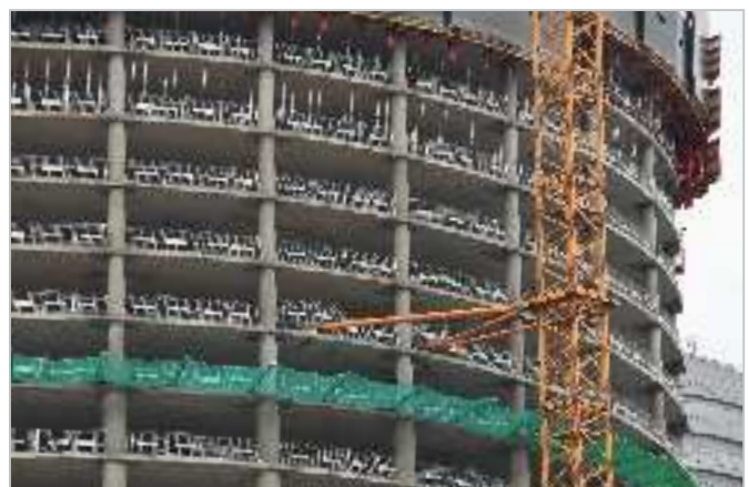
The use of safety nets for the construction of a skyscraper
