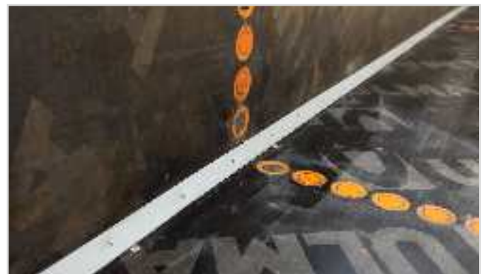
The chambering strips mounted inside the formwork
