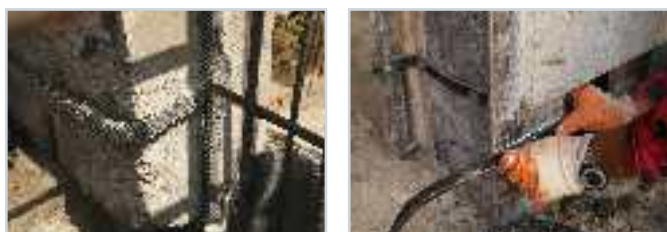
Example of use FORBENT tape type S
