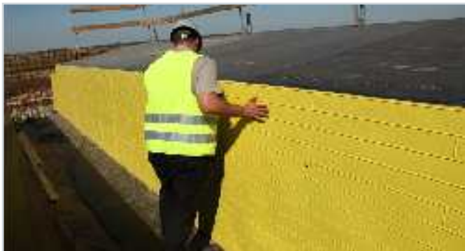
Control arrangement of the formwork mat
