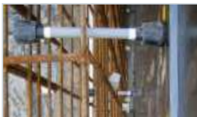
Using of the articulated nut KP-S B15
