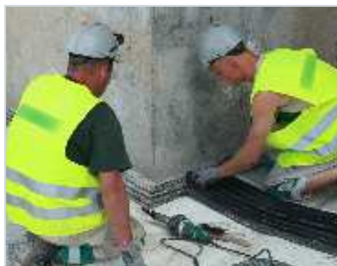
Mounting of sealing, construction of transport hub
