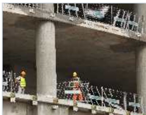
Installation of protective nets, construction of Warsaw Spire
