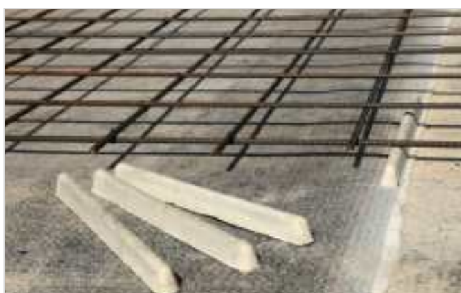
Using of concrete linear spacers
