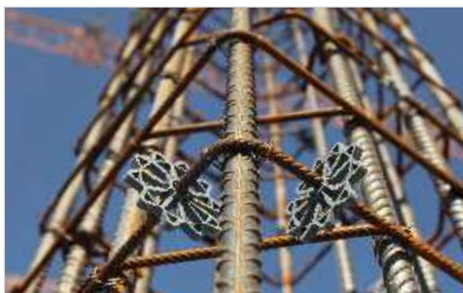
Using of point spacers PADIX
