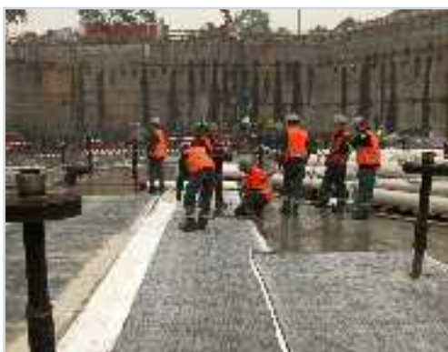
Mounting of sealing, construction The Second World War in Gdańsk
