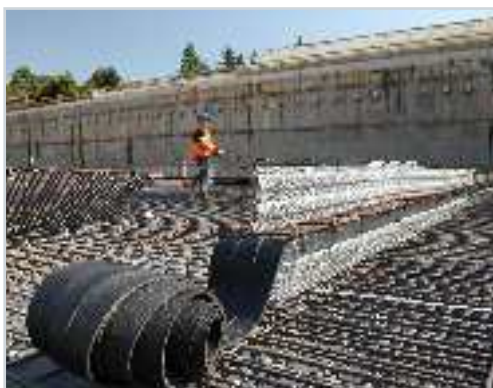
Mounting of sealing, construction Castle gallery in Lublin
