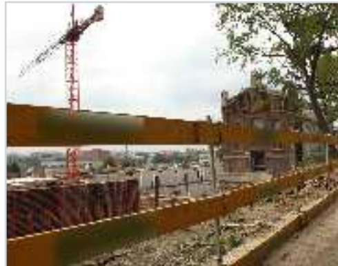
SECUMAX system, construction of the museum in Katowice
