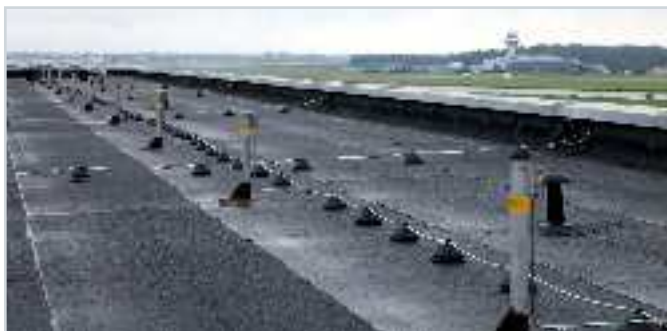
The SECUMAX INDIVIDUAL elements on the roof of the parking
