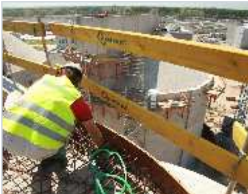
Mounting of sealing, treatment plant in Warsaw
