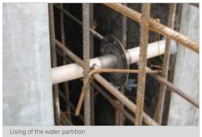
Transition to tie bar with distance pipe
